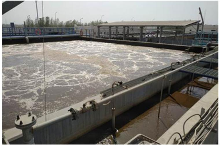
Retrofitted Aeration tank and post Anoxic denitrifying reactor with AC 920 biocarriers
