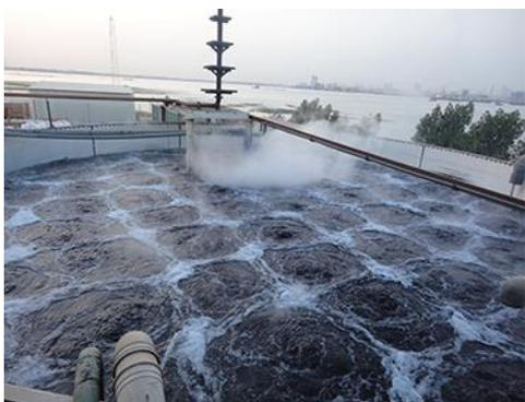
*Equalization tank with pH correction and color removal*
