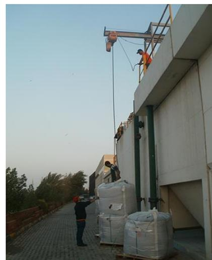
*Active Cell 920 media loading into reactor*
