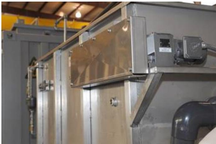
The DAF separates the solids from the bioreactor effluent.
