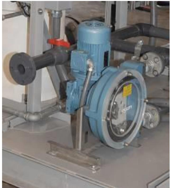
The peristaltic secondary solids pump transfers the solids removed in the DAF to the bioresidue storage tank.
