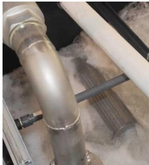
Effluent screens, or sieves, keep the Headworks Bio ActiveCell media in the reactor, while allowing the effluent to pass through.
