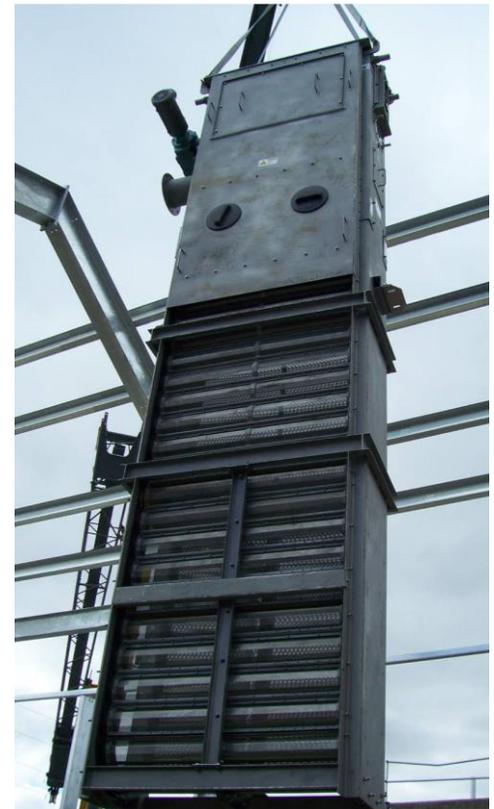
*Installation of Eliminator Band Screen by crane*
