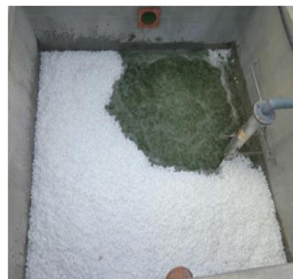
*MBBR tank (16 m³) loaded with a 44 % fill fraction of ActiveCell media*
