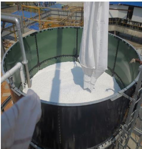
*Installation of Headworks ActiveCell mobile biofilm carriers to support very high concentration of attached biomass*
