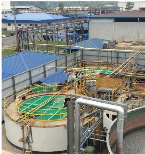
*Existing two stage active sludge process (ASP)*
