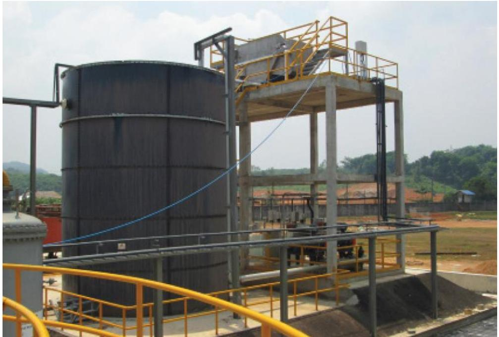
*Headworks BIO's Inc. roughing reactor based on moving bed biofilm reactor (MBBR) – MBBR is a self-sustaining biological process, eliminating the need to periodically waste sludge and the requirement to supply a dilute return activated sludge*
