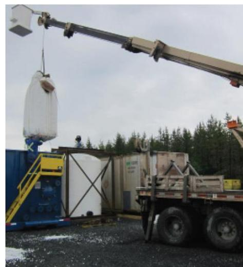
Seabee FRAC tanks being loaded with ActiveCell® AC<sub>920</sub> media
