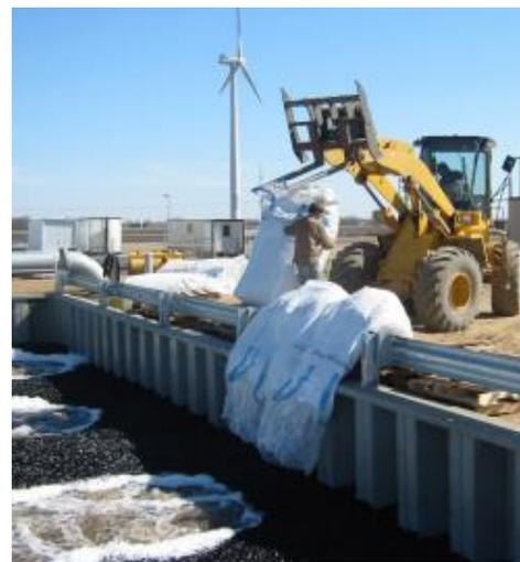
*Installation of ActiveCell media into the Moorhead WPCF nitrification reactor.*
