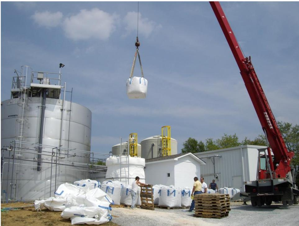
*Installation of the ActiveCell media by crane*
