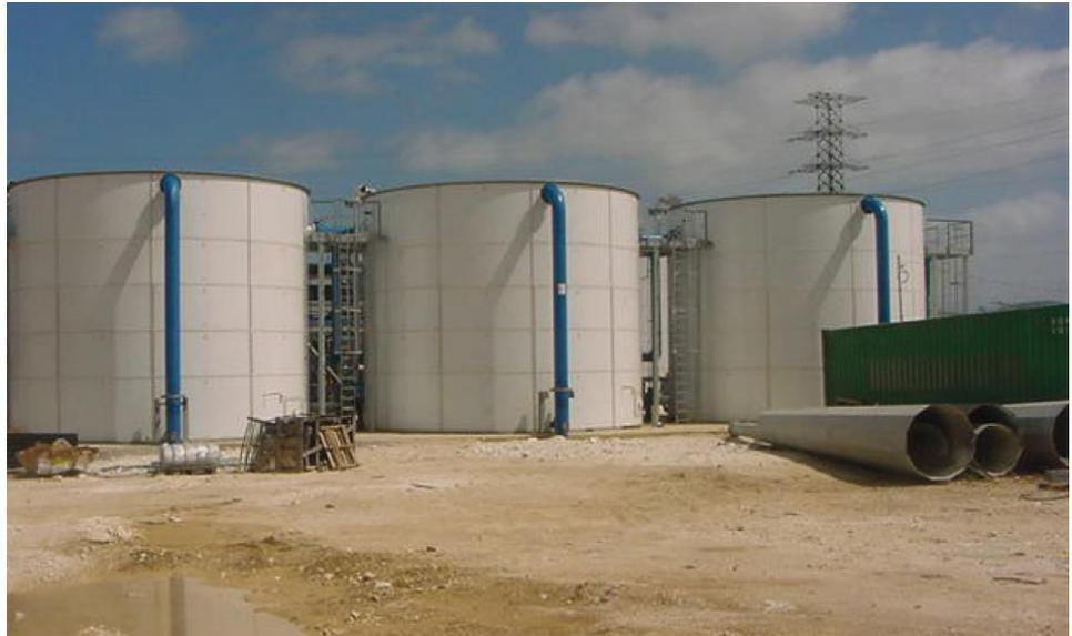
*Three-stage ActiveCell bioreactors to treat a wastewater flow of 1.8 MGD, resulting in reduced BOD, ammonia and TSS levels.*
