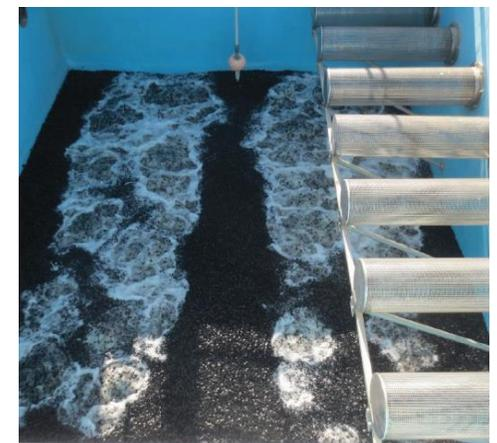
*The biomedium operates in a mixed motion with an aerated wastewater treatment basin.*
