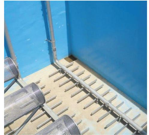
*Diffusers and aeration grids supplied by Headworks BIO Inc.*
