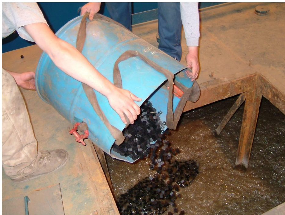
Installation of ActiveCell media into the nitrification reactor.
