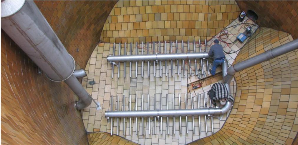
The bioreactor and related aeration system were installed in an existing stock tank. The tank was constructed of chemical and abrasion resistant tile-lined concrete, furnished with a heeled bottom.
