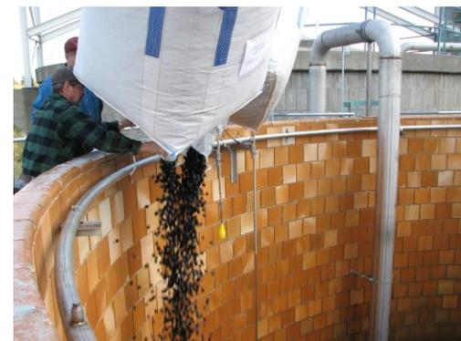
The 117,000 gallon bioreactor is loaded with a 67 % fill fraction of ActiveCell<sub>450</sub> media.
