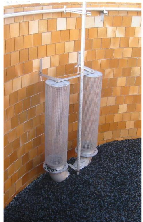
*The treated wastewater is pumped from the bioreactor via an internal retention screen riser mounted vertically to minimize air entrainment and to allow maximum wastewater retention with the bioreactor.*
