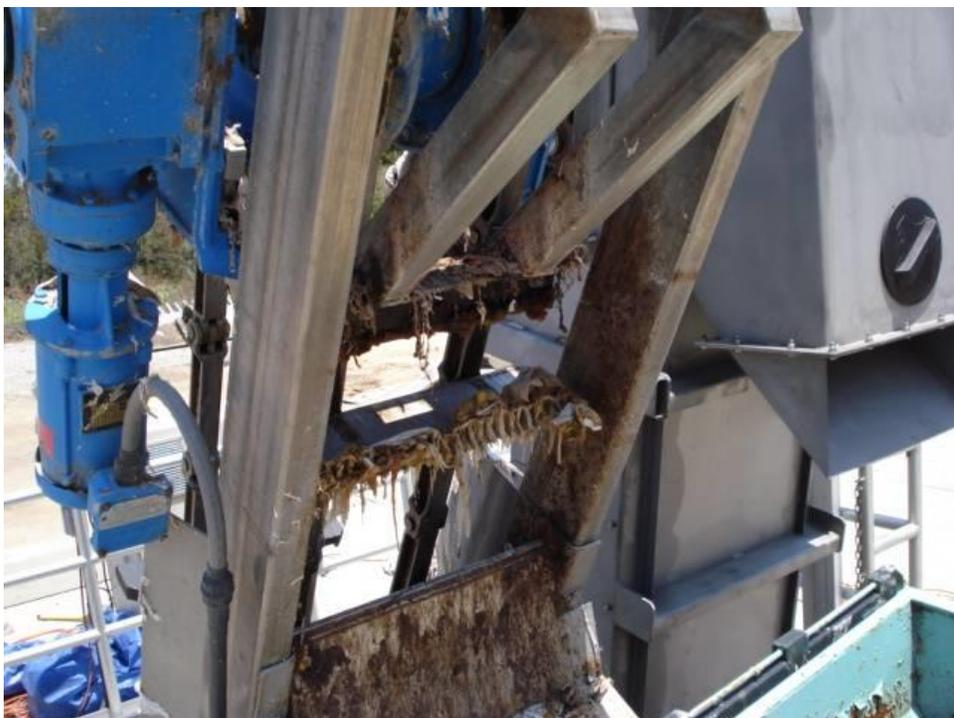
*Debris collected on the old screen's chains and scraper mechanisms that frequently required cleaning*
