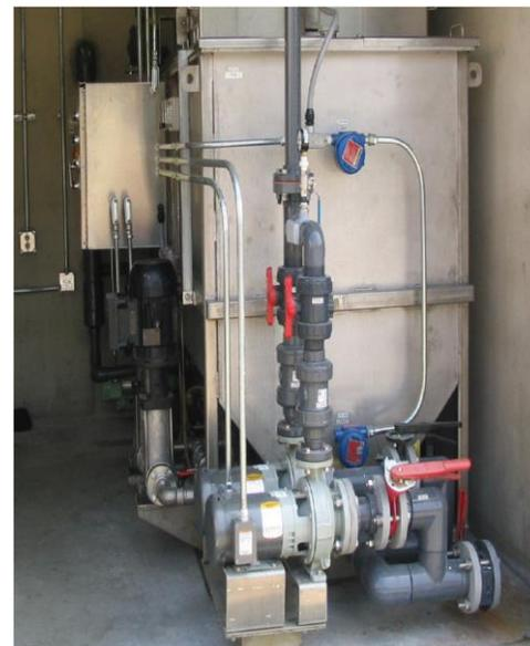
*The process stream is pumped at a controlled rate to a pre-dissolved air flotation (DAF) system.*
