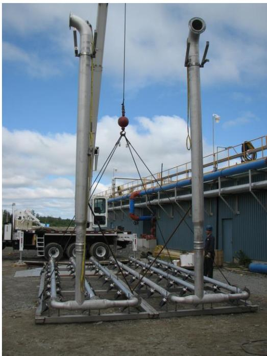
The aeration grid was mounted on a stainless steel support frame and then lifted into the basin by a crane.
