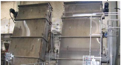
Purportedly the largest bar screens in the United States, the Headworks two (2) Mahr Bar screens, almost 70 feet in overall length, is installed in Mill Creek WWTP in Cincinnati, Ohio.
